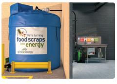
The energy rich slurry is stored on-site in a 3000-6000 gallon tank until hauler transports to AD facility.
